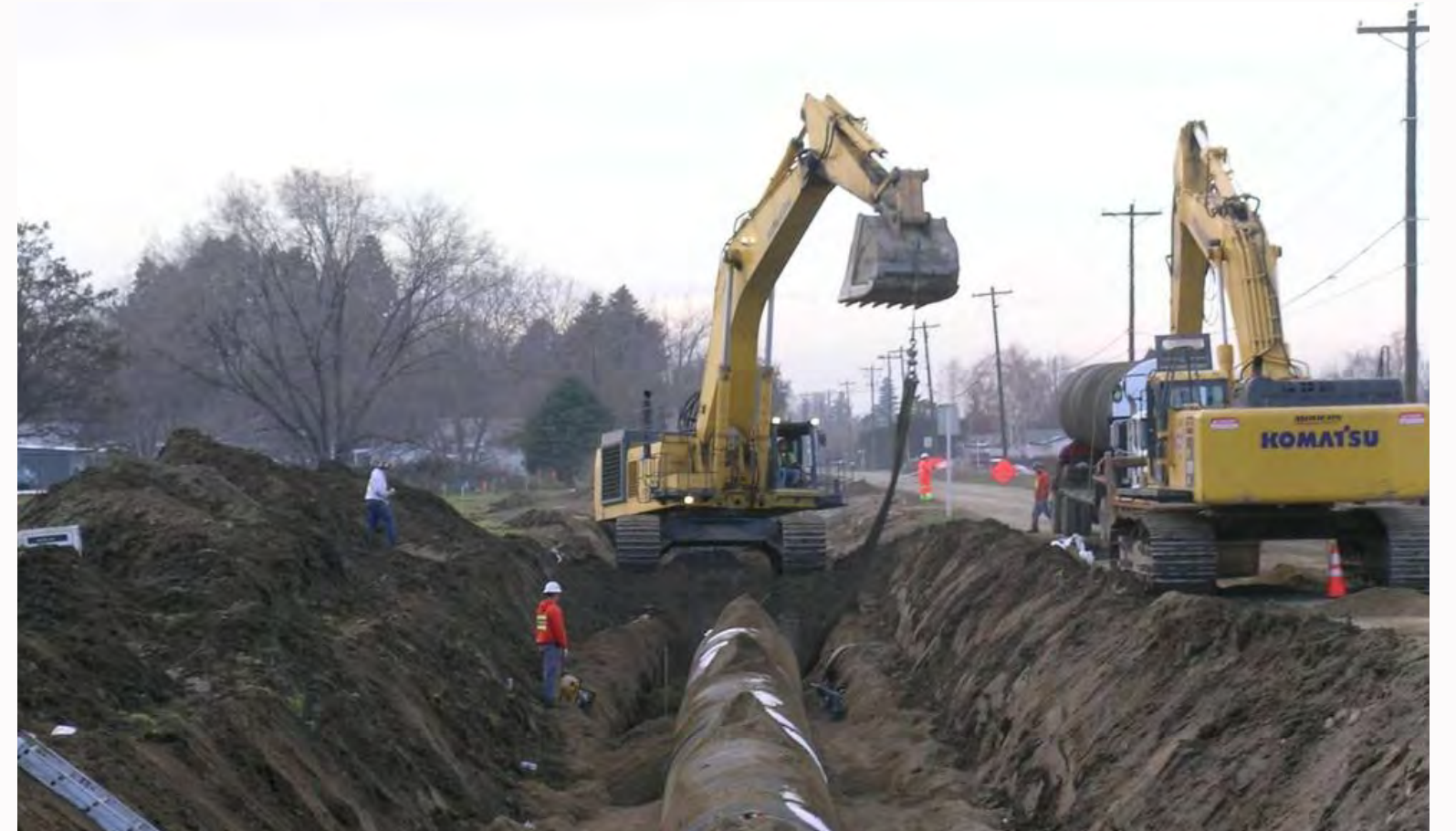
Enclosing open canals
