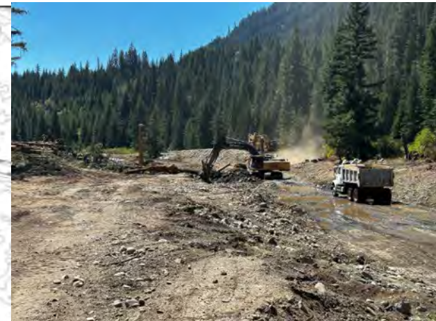
Side channel excavation
