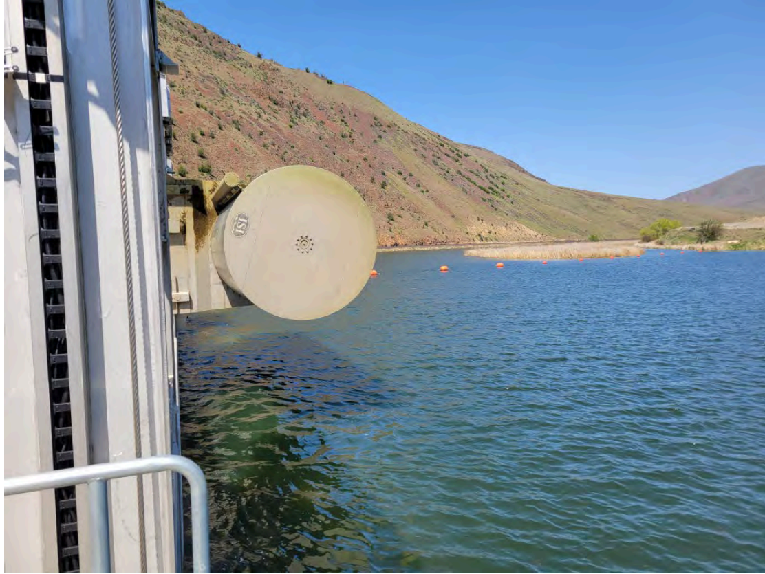
New fish screens (out of the water)
