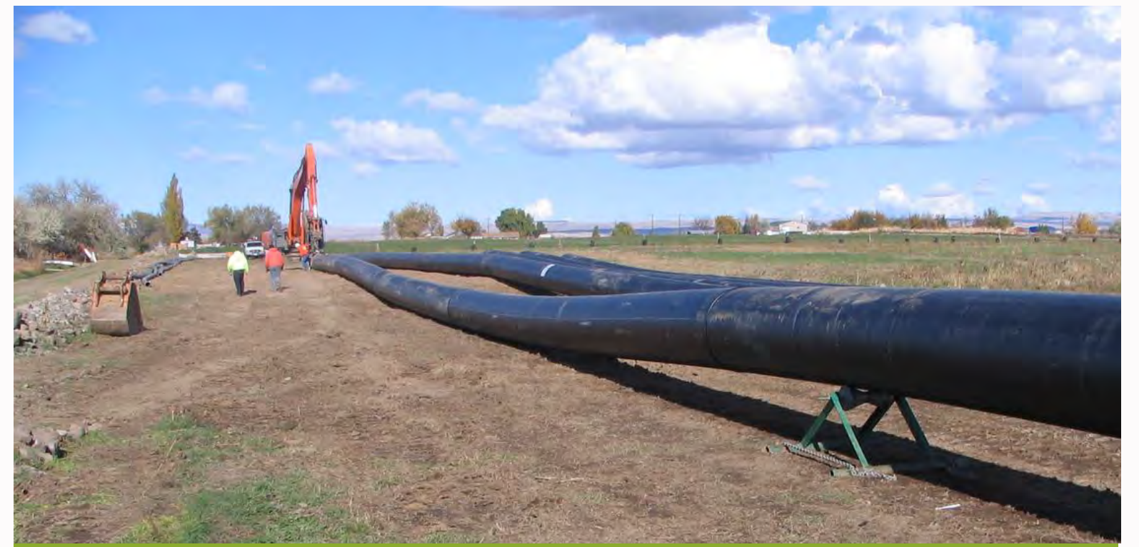
HDPE Pipe installation
