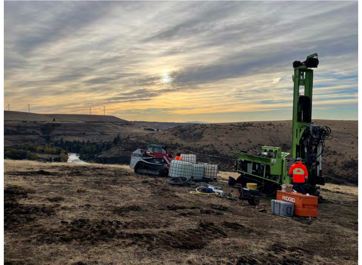
Geotech drilling at Springwood, Fall 2025 Photo by Jacobs Engineering
